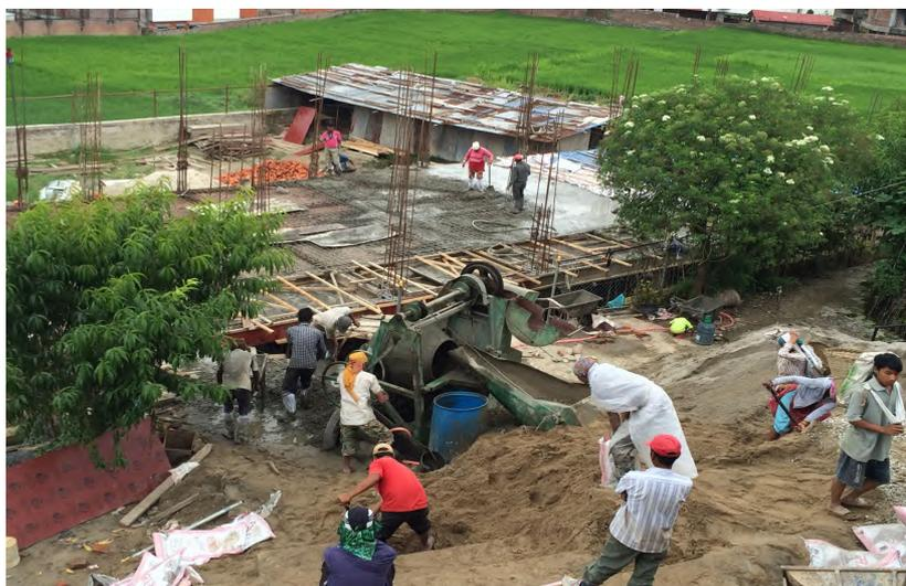
The highlight for this month was the casting of the slab over the ground floor. It took over 10 hours with over 30 labourers working with only a little break to have food prepared for them by Tewa. The day was cloudy with no rain – this made it easy for the workers and ensured the slab
